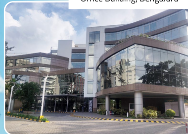
Office Building, Bengaluru
